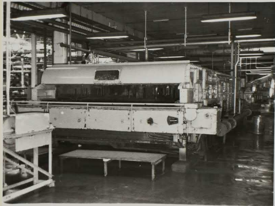
No..5 line. Pasteuriser
