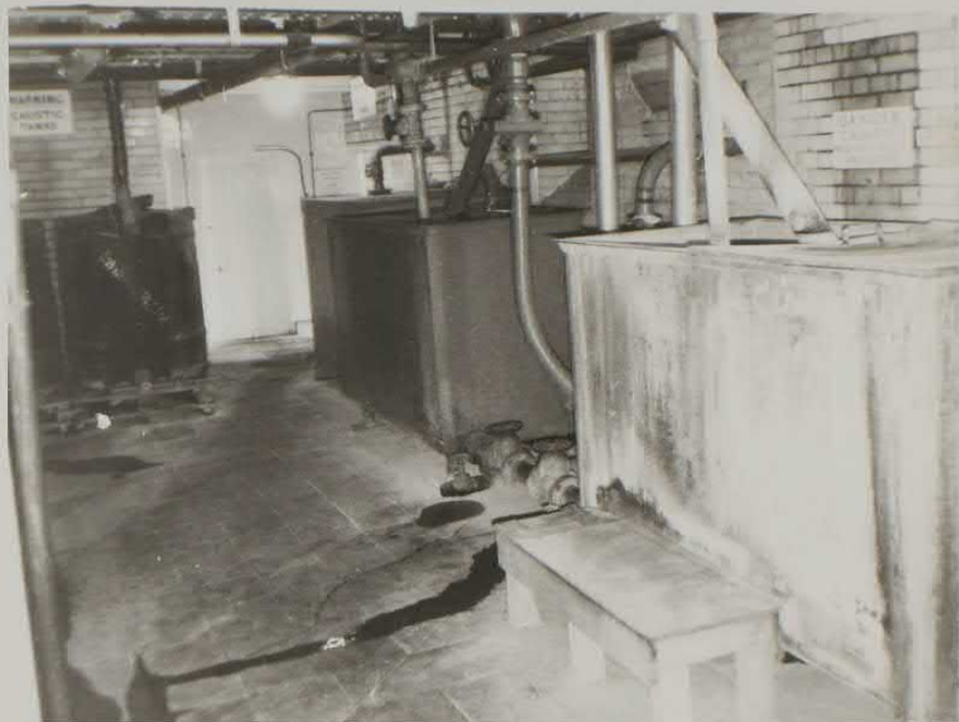
Caustic tanks near underbacks
