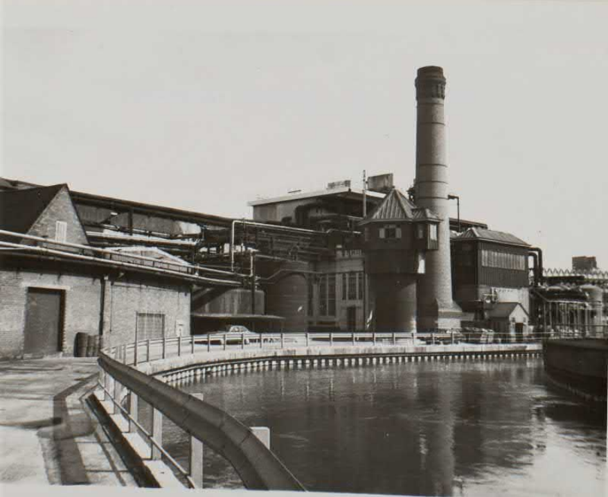
External of Power House 1979
