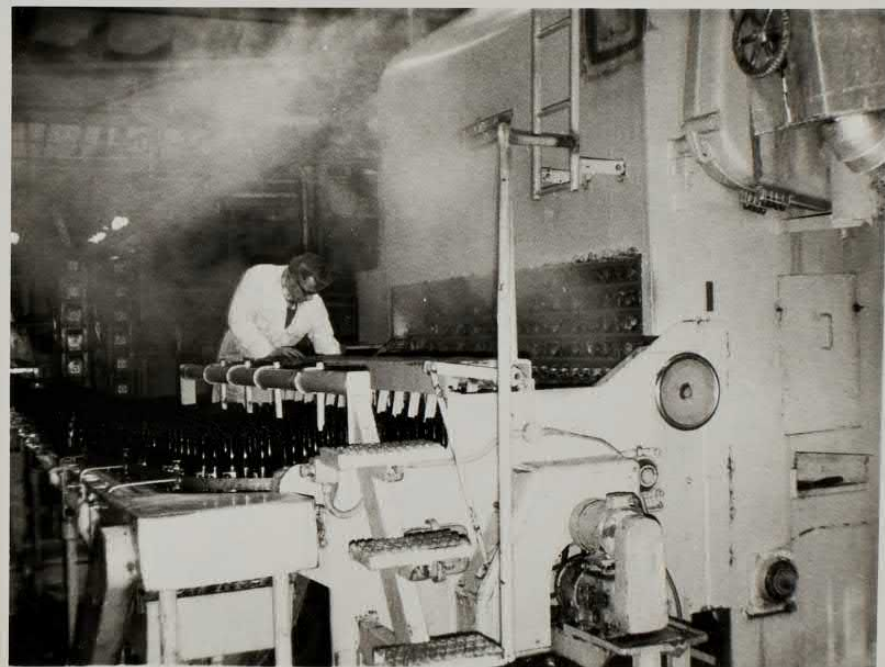
No.1 line bottle washing machine, inlet end
