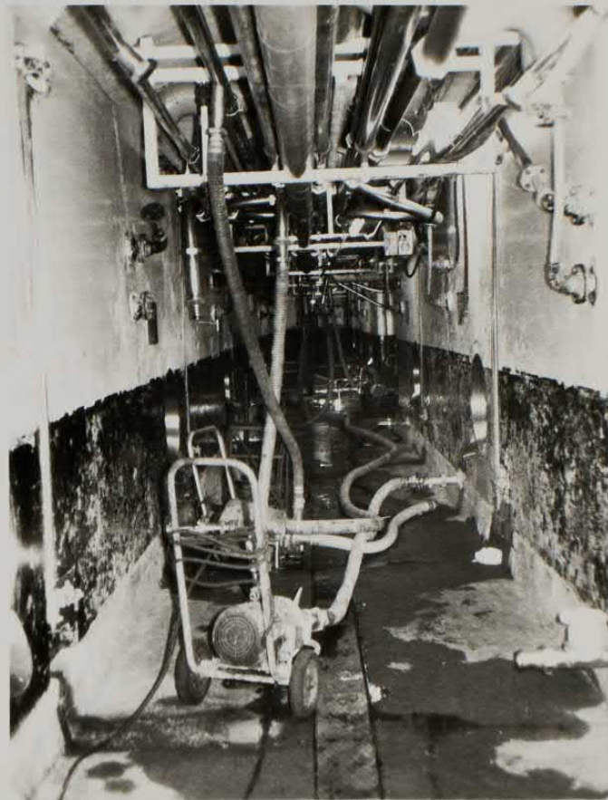
Concrete beer storage tanks (lined)
