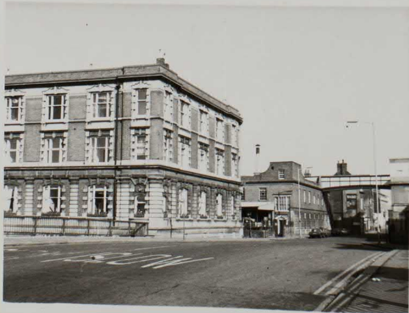
Looking up Bridge Street towards town 1979 Office block on left.
