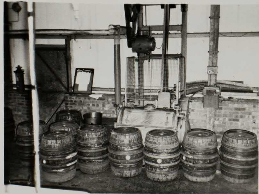
Washing machine for temporary shives
