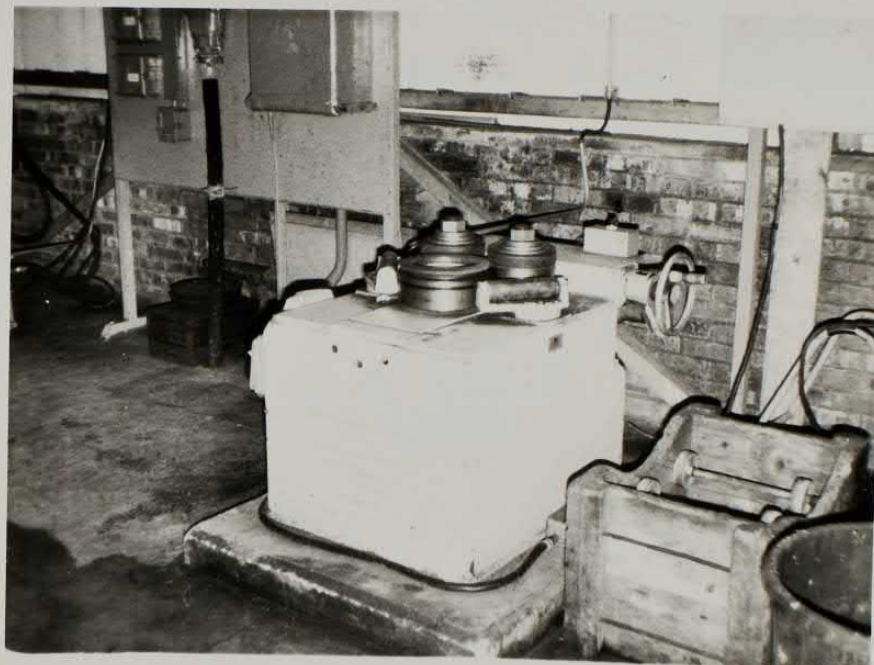
Cask spinning machine for cask repair
