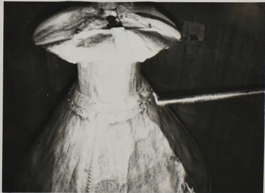
Casing over steam heater inside wort copper No1.
