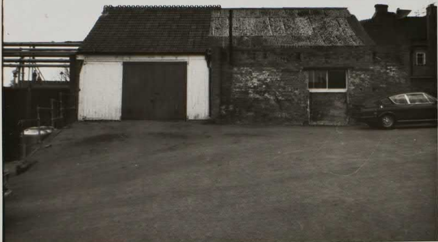
Rear of Castle Street. Remains of old South Berks Brewery with cellars underneath 1979
