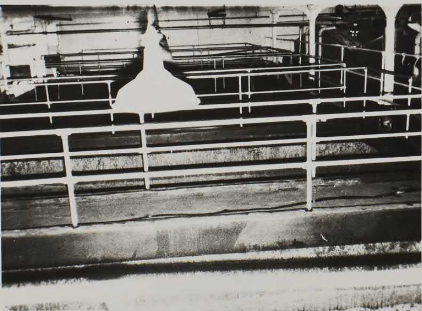
The bitumin lined concrete fermenters
