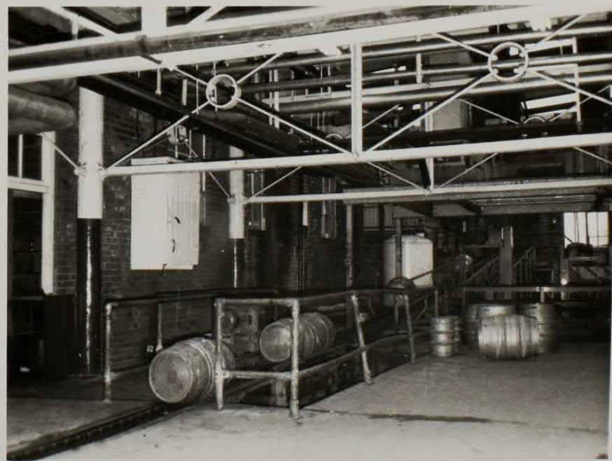
Conveyor for casks from washer to filling lines (looking back)
