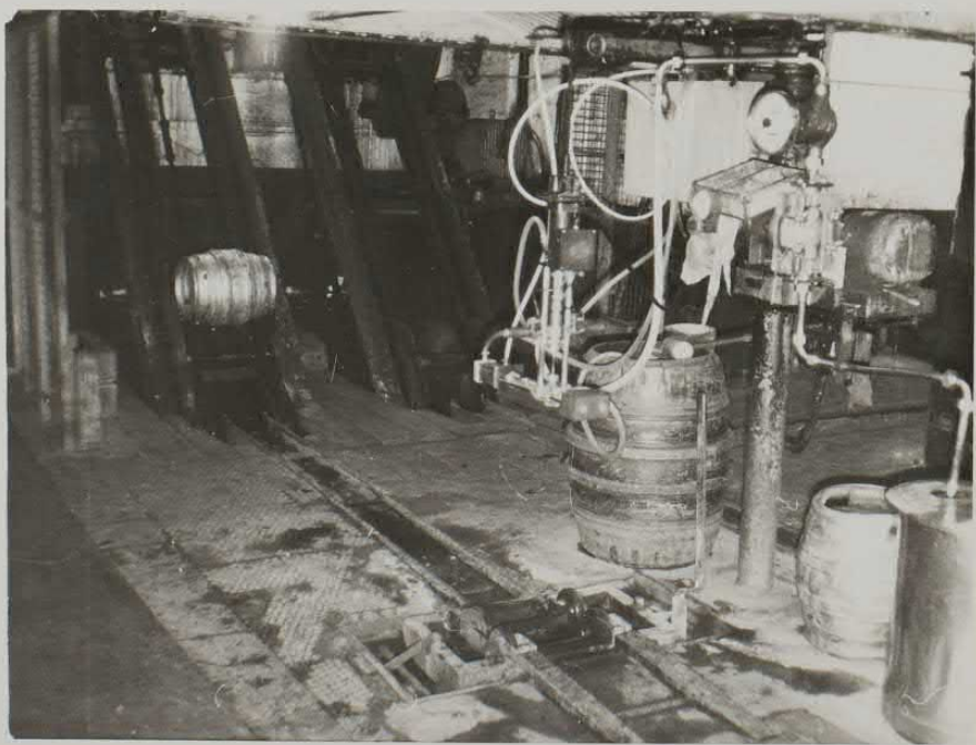
Cask fining machine and cask elevators
