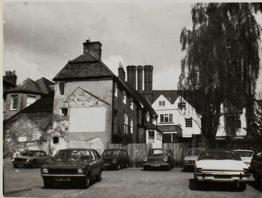
Rear of 17 Castle Street 1979
