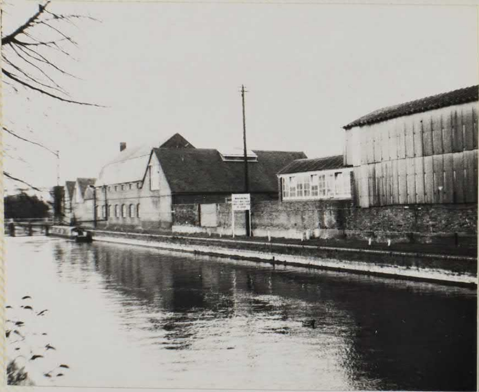
Looking up River Kennet from Bridge Street 1979
