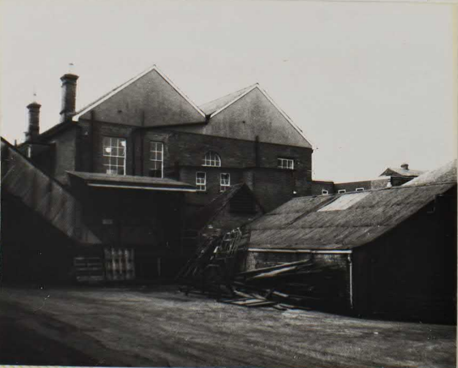
Rear of Seven Bridges House 1979
