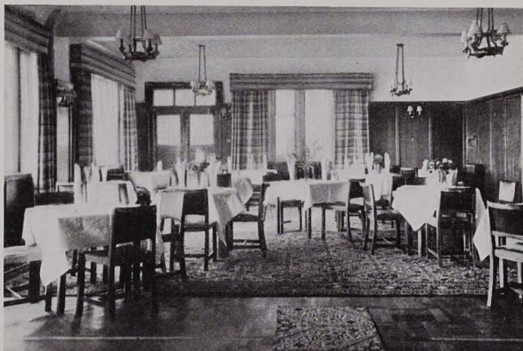
Restaurant, showing doors to Gardens and Car Park at rear
